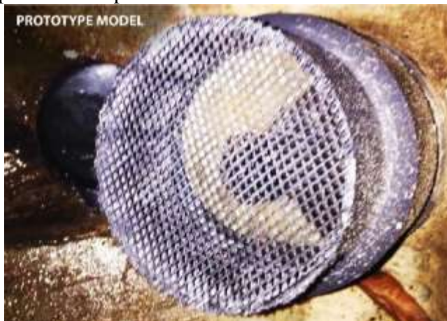
Figure 5: Prototype design of interceptor gully trap
